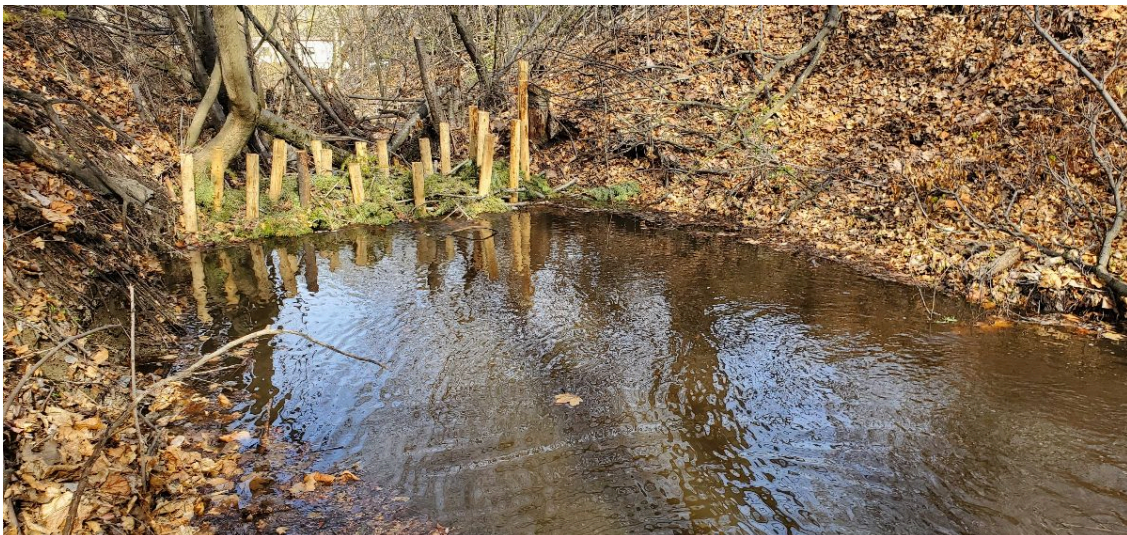
The completed BDA with fir boughs woven into posts to capture sediment traveling in the stream that then fills gaps in the BDA and slows water even more.
