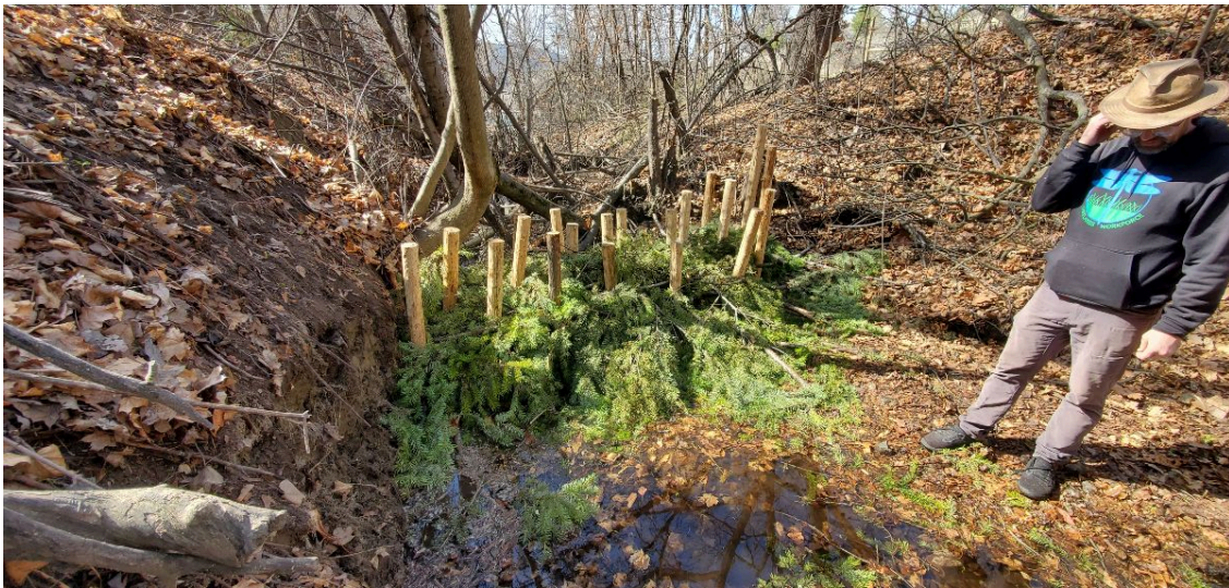
The completed BDA with fir boughs woven into posts to capture sediment traveling in the stream that then fills gaps in the BDA and slows water even more.
