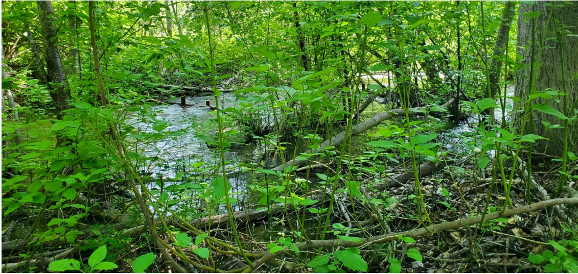
First High Flow event after installation - May 2021
