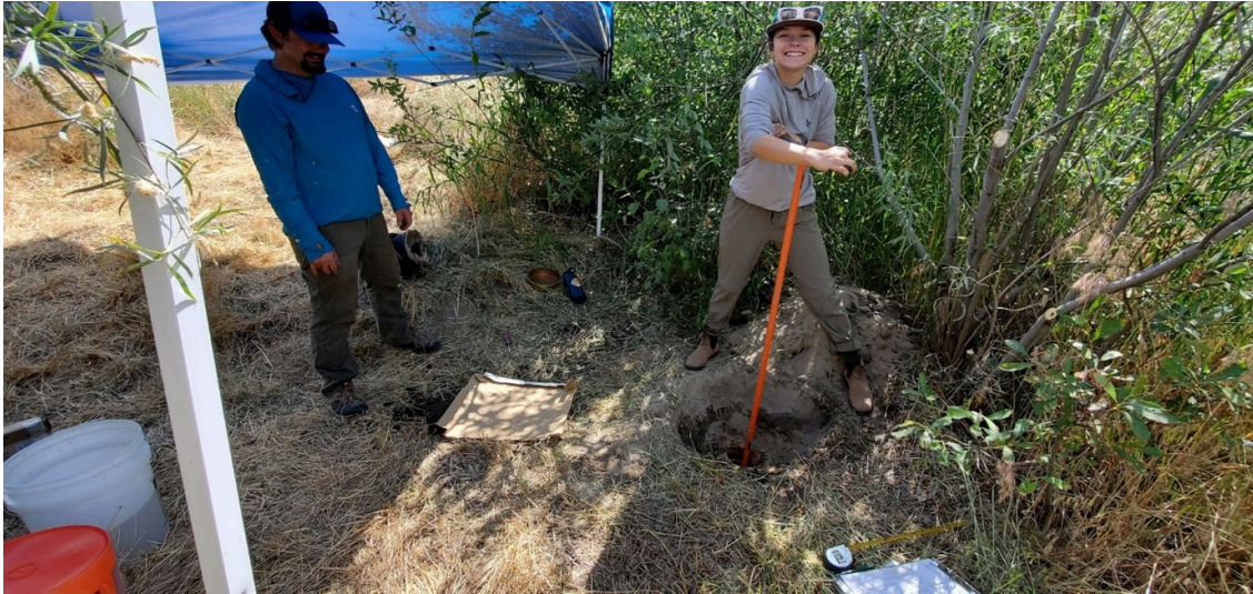
Working hard digging a ground water well.
