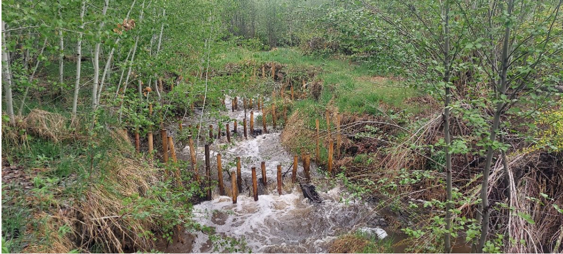
Photo: April 2023 Chiliwist Creek with her new BDA's slowing water and capturing sediment
